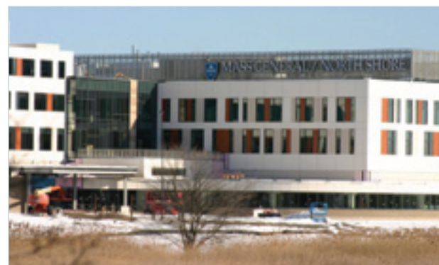
Exterior of Outpatient Care Center, Danvers, Mass.
